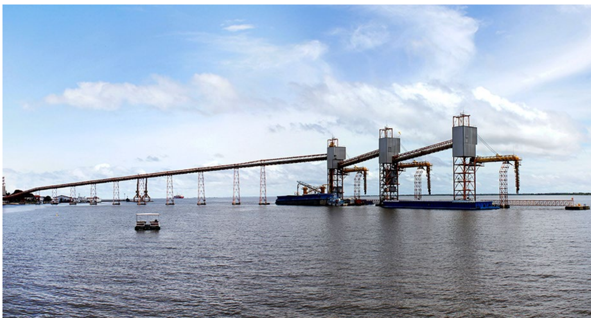
A Conveyor belt feeding hoppers as a soy export terminal owned by Cargill. Tarcisio Schnaider / IStock
