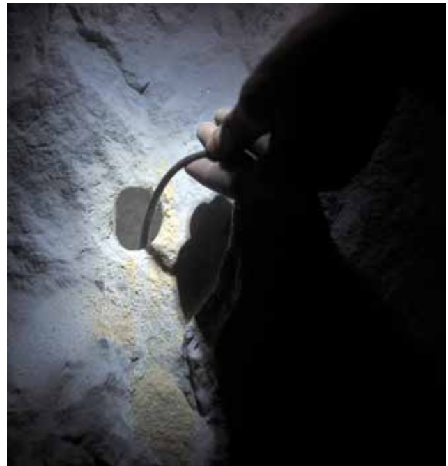
Dynamite in place before blasting
